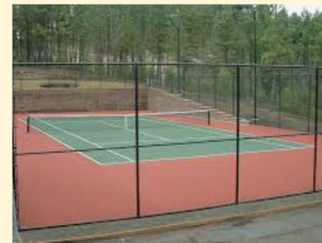
Tennis Court Fence
